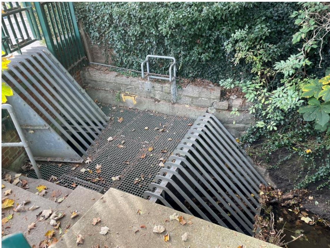
Photo 7 – Eastwood Brook trash screen at corner of Glenwood Avenue
