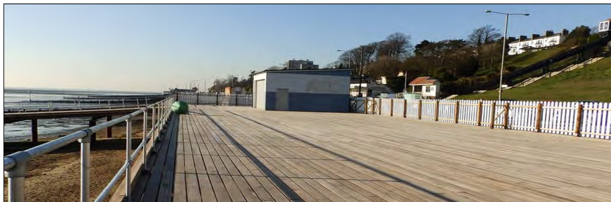
Figure 9.2: Alexandra Yacht Club new facilities opened in 2017
