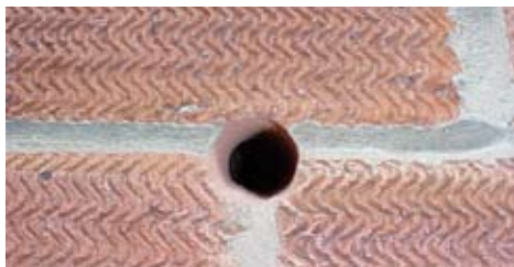
An injection hole prior to filling
