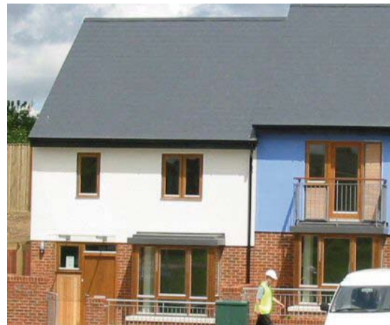
Oakridge development – light gauge steel frame panellised construction (photo courtesy Sentinel Housing Group)
