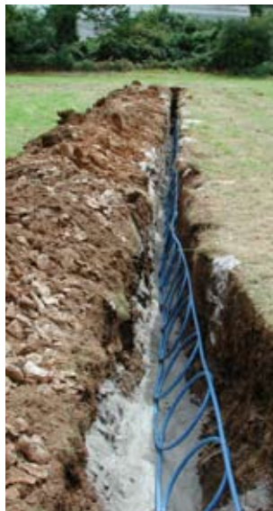
A ground-source heat pump
