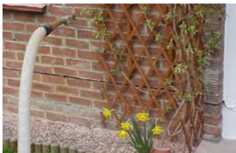
Insulation being injected into the wall
