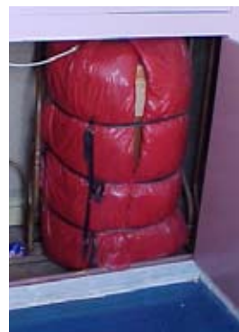
A well insulated cylinder jacket
