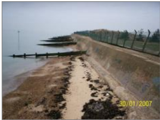
Partial view of work site
