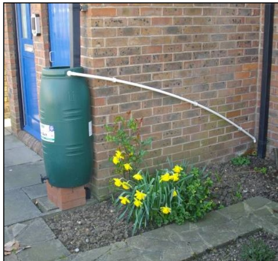
Figure 10-2: Example of water butt in use
