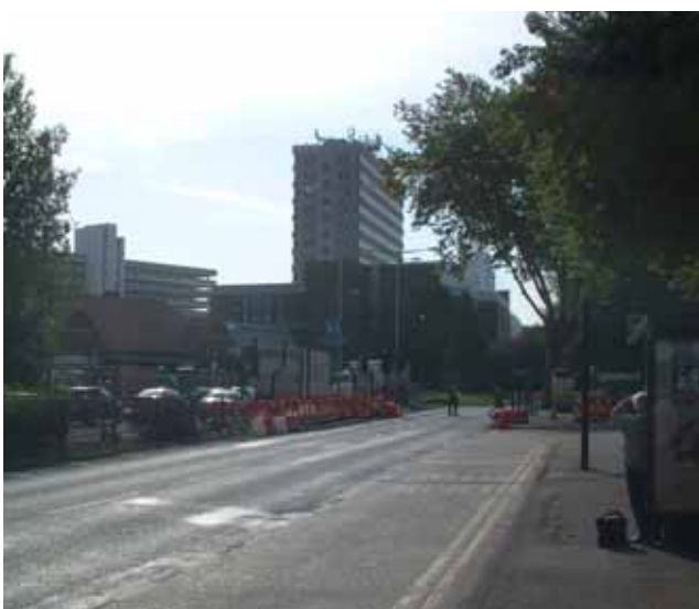
Victoria Avenue as it exists now
