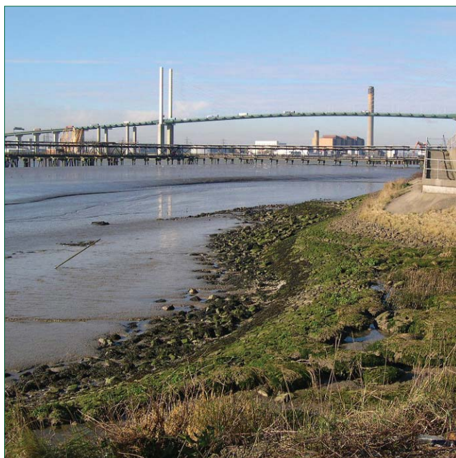
Existing strategic landmark - Queen Elizabeth II Bridge
