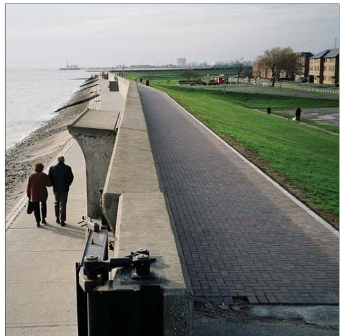
Sea wall at Canvey Island
