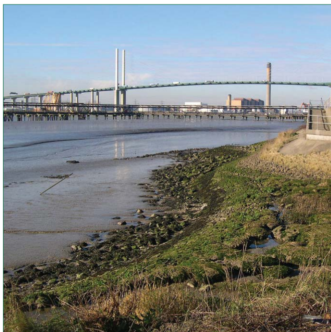
Existing strategic landmark - Queen Elizabeth II Bridge
