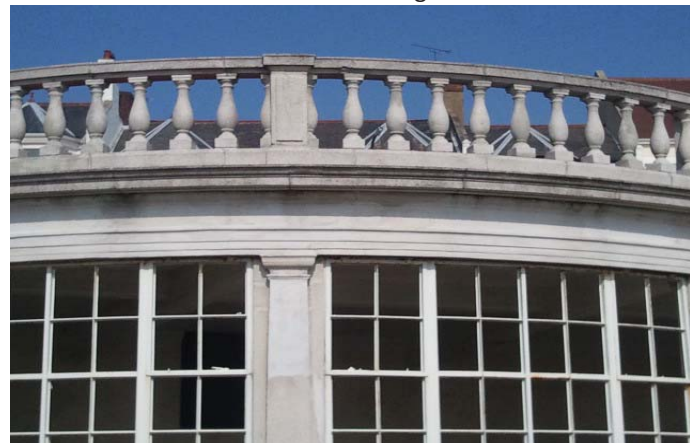
The Sun Shelter's windows and terrace
