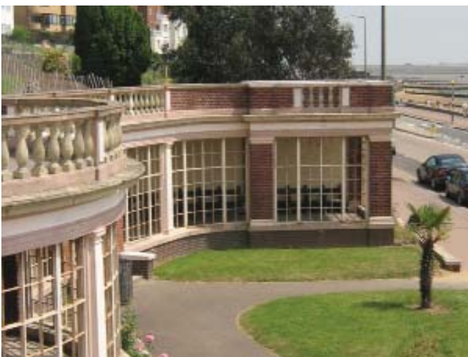
The Shelter looking east
