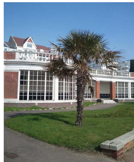
View of the Shelter
