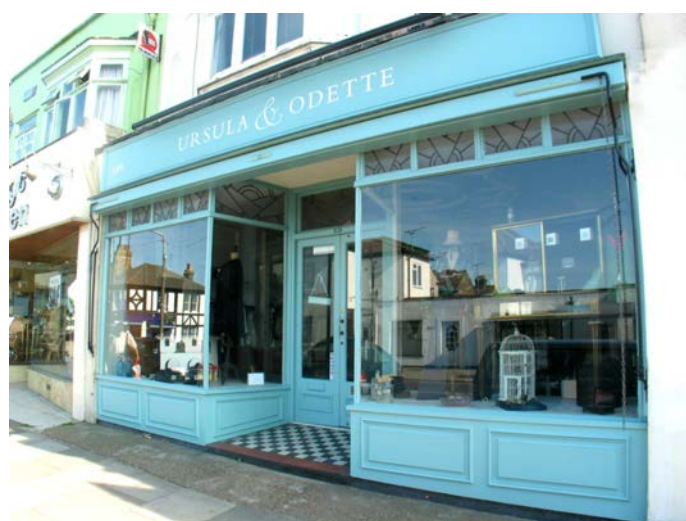
A traditional shopfront in Leigh includes decorative fanlights, stall riser & a recessed doorway.
