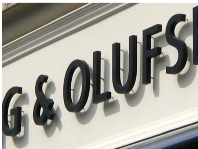
Raised letters can give extra depth & articulation to a fascia sign.
