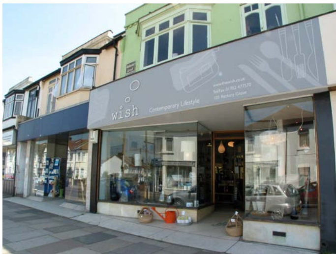
A modern shopfront in Rectory Grove is a simple yet interesting and well articulated design.
