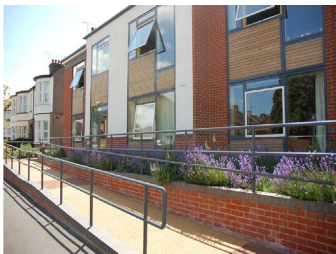
This access ramp has been designed to incorporate the same materials as the main building and a significant area for landscaping.
