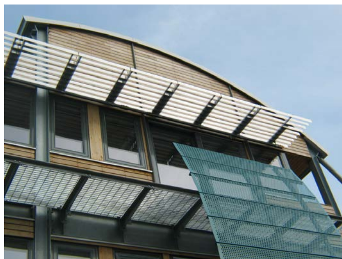
The solar shading & privacy screens on this surgery are an important part of the buildings character, but also serve to make the building more comfortable for its users.
