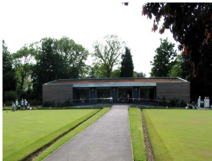
The green roof at the bowls pavilion at Priory Park will significantly reduce the surface water run off the building.
