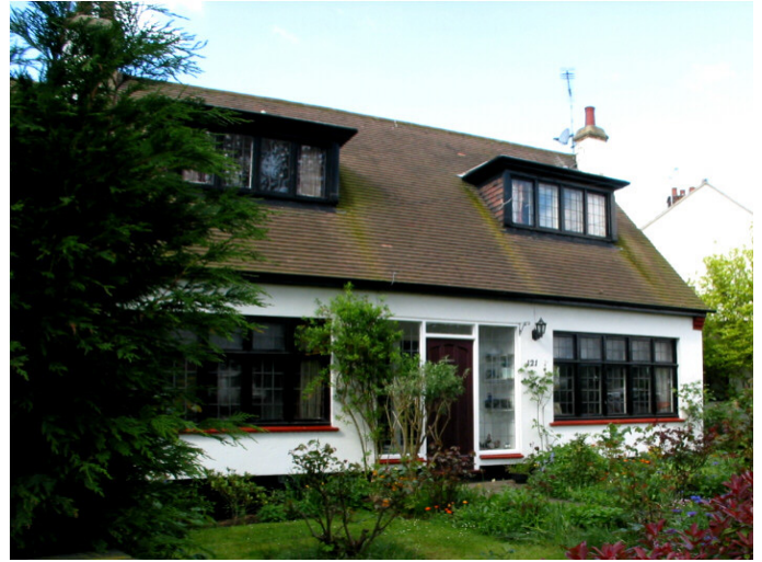
The dormers on this chalet in Thorpe Bay draws reference from the ground floor windows in their design and alignment but are subservient in scale
