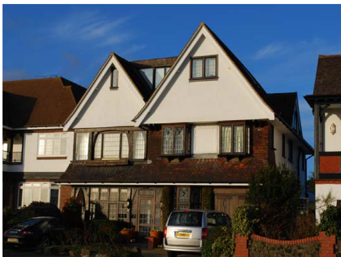
A clever yet subtle roof accommodation intervention along Chalkwell Esplanade.
