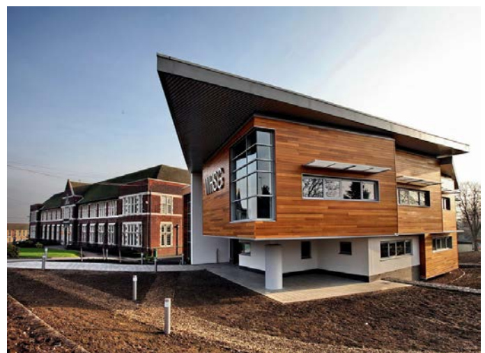
Extension to Westcliff High School for Girls contrasts effectively with the traditional school building.
