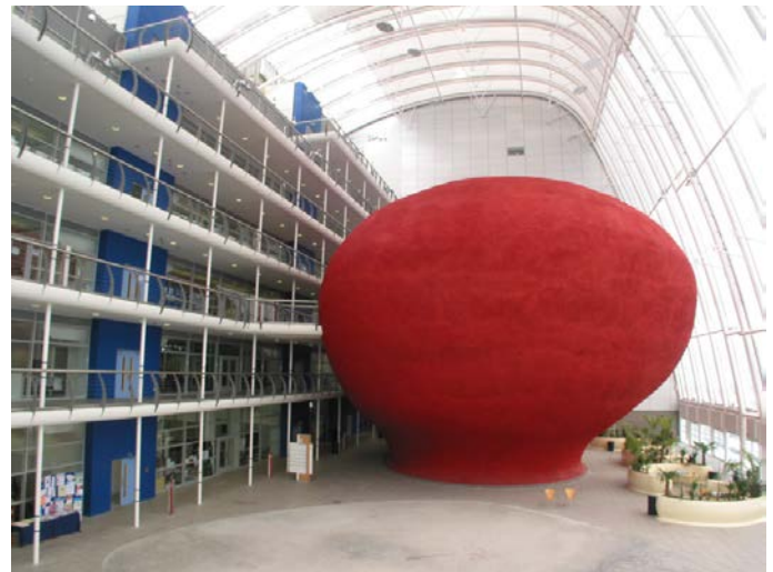
The atrium and pod of the South East Essex College provides a stimulating learning environment for students.
