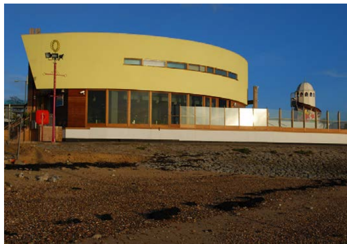
The Southend Radio station building forms a new vibrant landmark on the Seafront.
