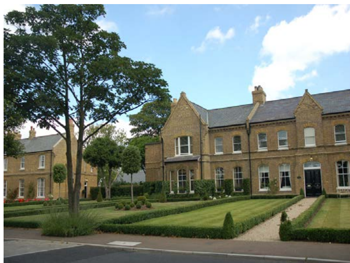
Refurbished listed buildings at Shoebury Garrison.
