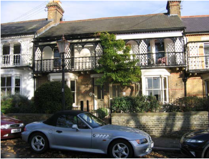
Typical housing in Leigh Conservation Area where decorative balcony detailing is a common feature.
