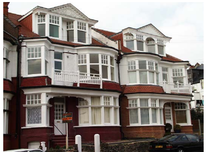
Traditional development in conservation area's in particular should take extra care to exactly match the detailing of the original buildings. The new building on the right is a replica of its neighbour in Palmeira Avenue.
