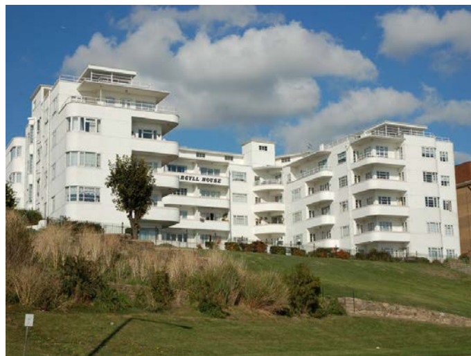
Argyll House a flatted block from the 1930's is an important seafront landmark and on the Council's local list.
