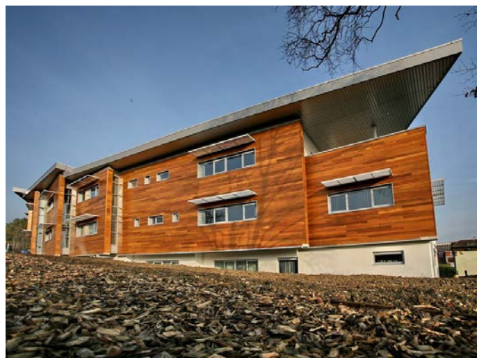
The high quality materials and detailing of this school extension in Westcliff contribute significantly to its success.
