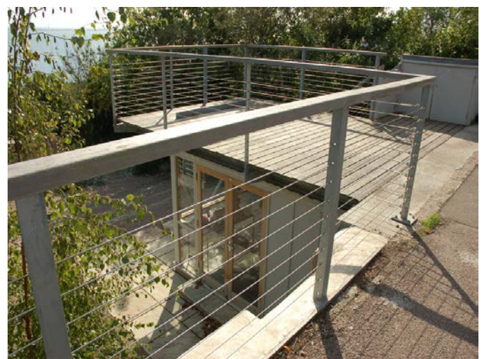
This forecourt parking area in Grand Parade for a property in Undercliff Gardens below has minimal impact on the street scene and allows public views across the site to the estuary.
