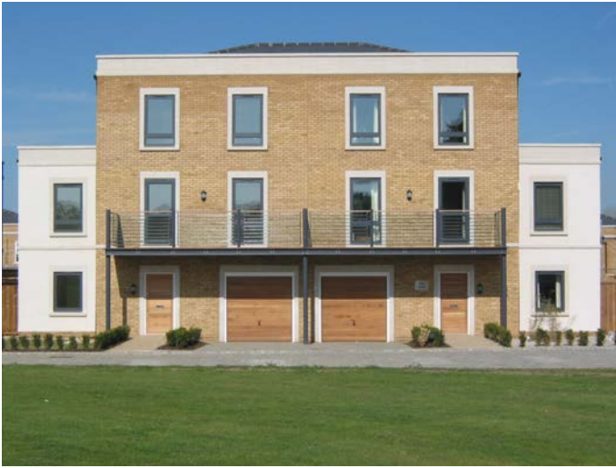
Garages and forecourt parking have been carefully integrated into these new town houses in Shoebury Garrison.
