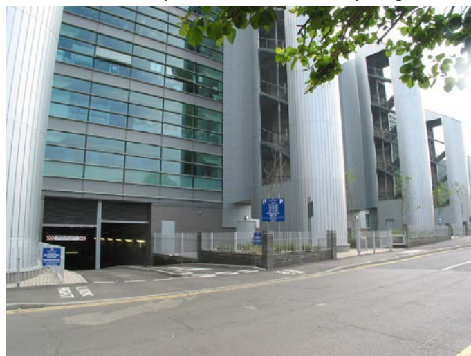
South East Essex College includes an underground car park which is safe & secure and has minimal impact in the streetscene.
