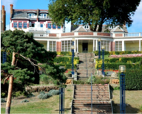
Large Edwardian sun shelter within clifftop gardens. Red brick with stone detailing and columns with parapet roof
