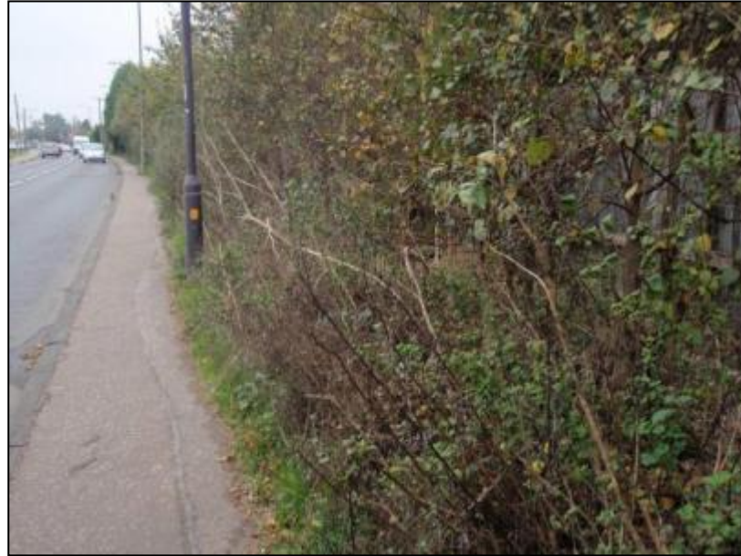
Figure 3.12 – Narrow footway on South End Road
