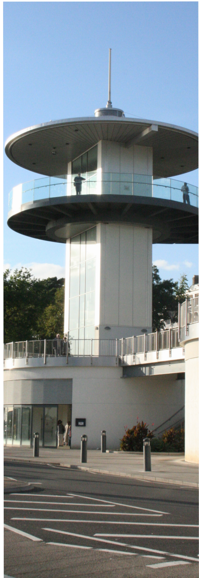
Regeneration of Pier Hill
